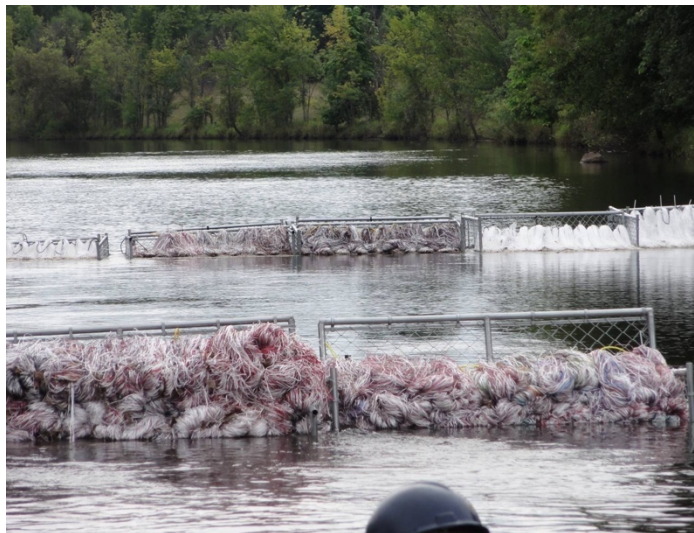
Figure 27 – Gabion baskets stuffed with viscous oil snares. Source: USEPA
