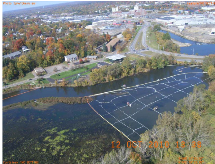
Figure 32 – Submerged oil recovery executed in pre-boomed cells. Source: USEPA
