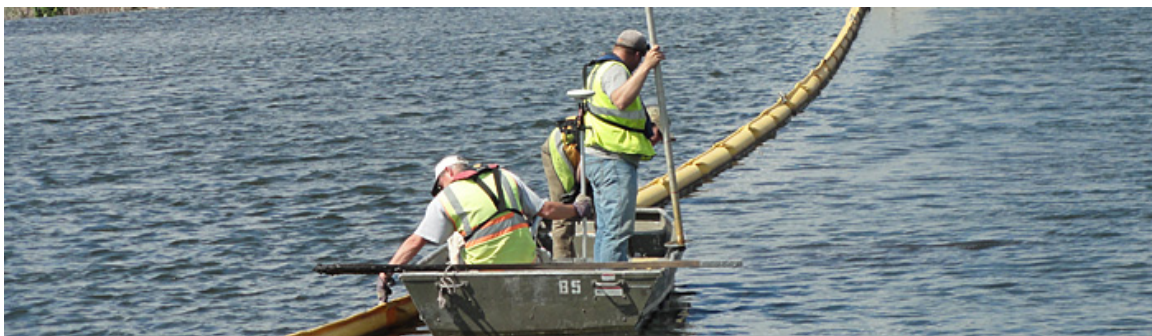
Figure 13 – Manual agitation to probe the bottom for submerged or sunken oil. Source: USEPA
