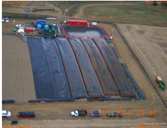
Figure 34 – In-situ treatment of dredge spoil water. Source: USEPA
