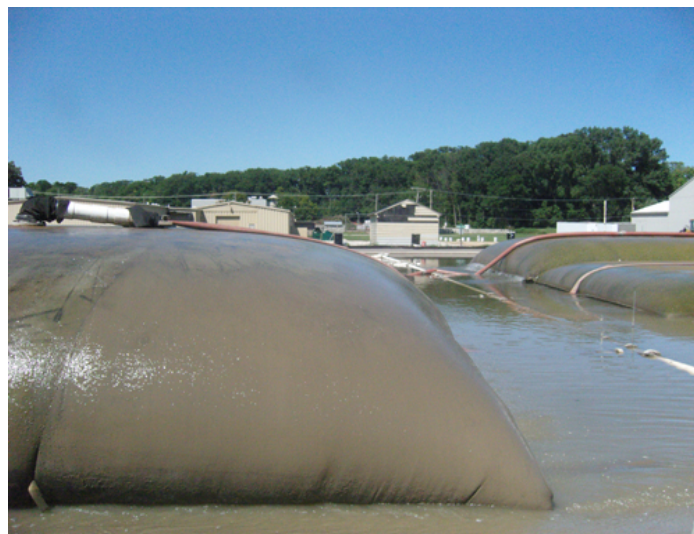
Figure 33 – Dredge spoils being dewatered through geotubes. Source: NOAA
